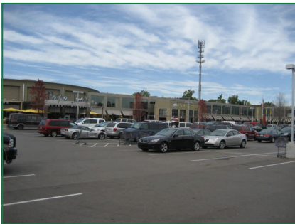
Photo Above: View new shopping center roofed by Royal Roofing Company.
