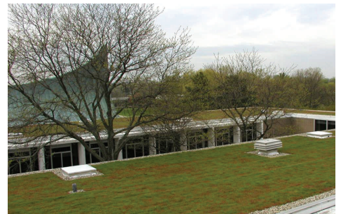
Photo Above: Sisters of Mercy Academy with New, Royal Roofing Installed, Green Roof System.
