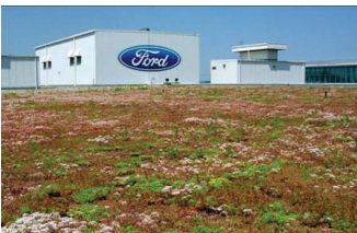
Photo Above: Green / Living Roof of Ford Rouge Plant—Dearborn Truck Final Assembly building. Green Roof System provided by Xero Flor America, LLC.
